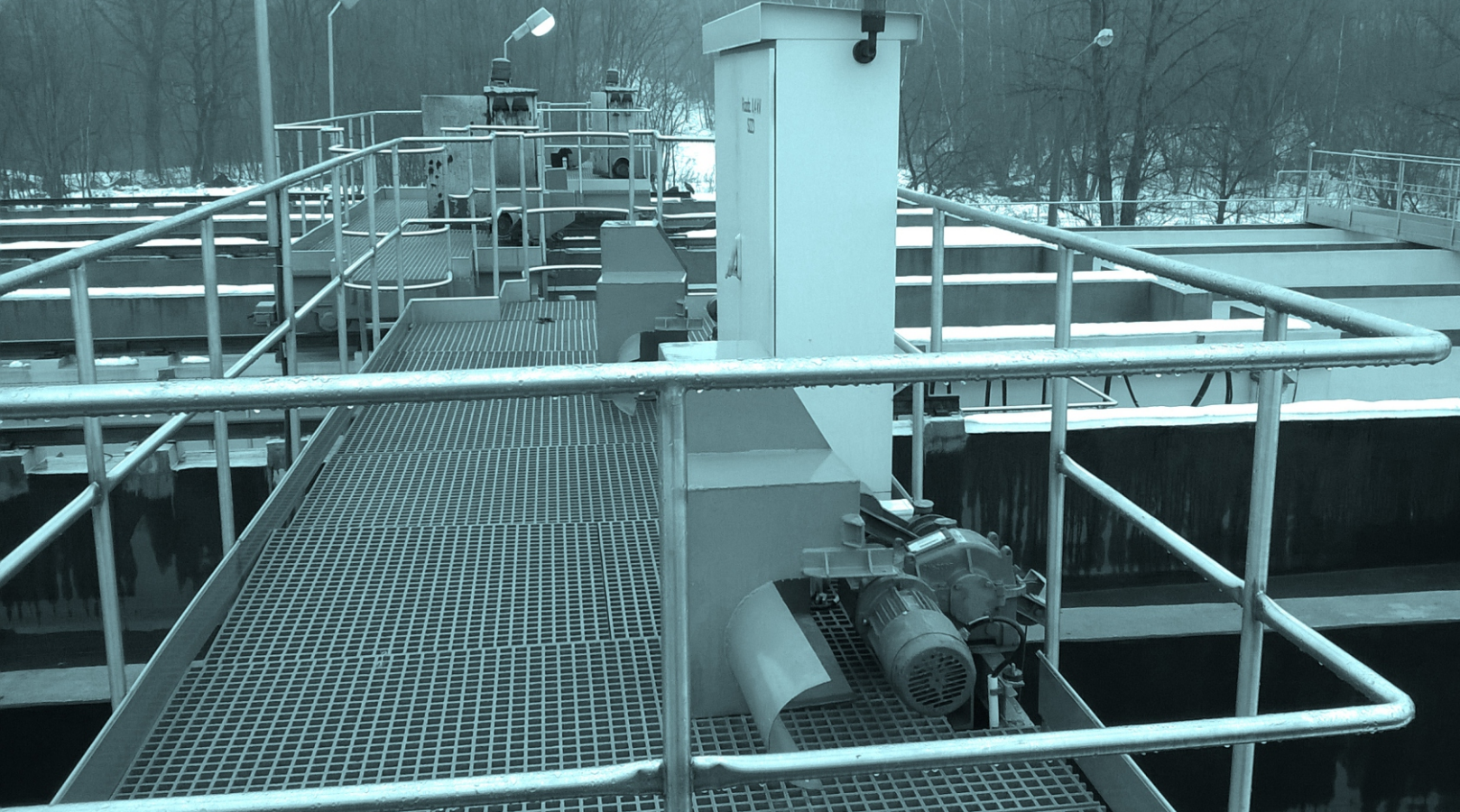
Sand scraper type ZGP
