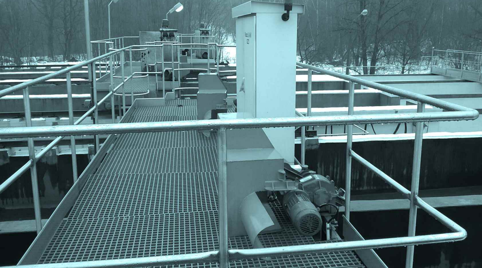
Sand scraper type ZGP
